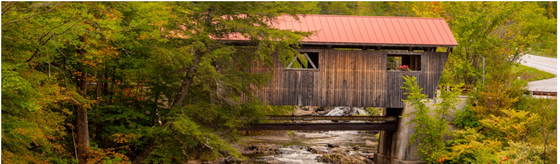
Johnson boasts an iconic covered bridge that sits above the Gihon River.
